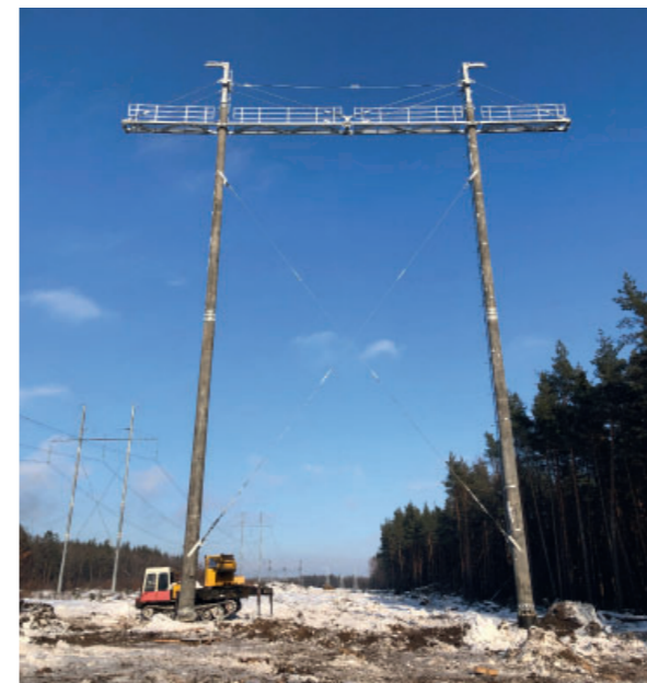
Fig. 3. 2SPB500-3V power transmission poles on 500 kV "Donskaya AES – Staryy Oskol 2" overhead line
