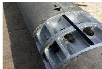
Fig. 1. Internal flange for connecting sections (typical solution)
